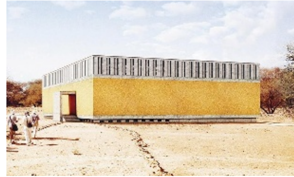
Two renderings of the Meroe Royal Baths Protective Shelter in Meroe, Sudan, an ancient city dating back to the first century AD and now listed as world heritage by UNESCO. The project provides a protective structure against wind and weather for the Royal Baths, and will be made with a thick wall of mud bricks to control internal humidity and natural ventilation.
